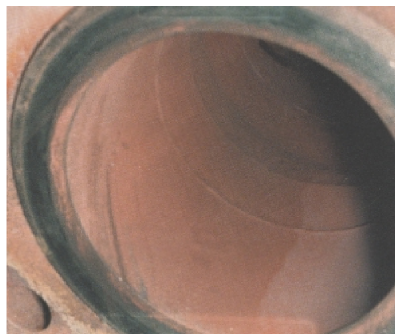
Conserved pipe section, protection effect after draining
